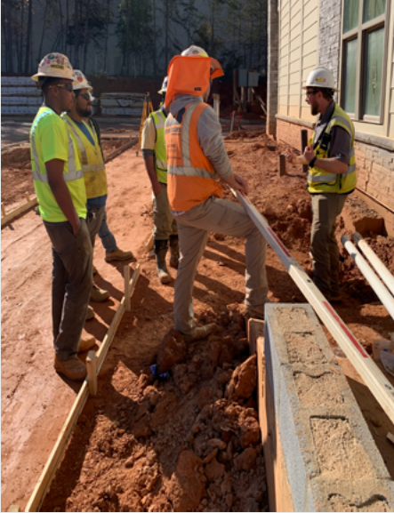
UC2 crew learning to calculate steps to match sidewalk landings prior to placing concrete
